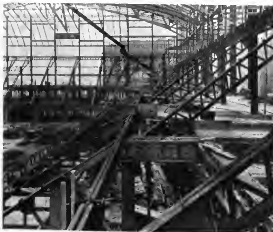
A SECTION OF THE BALCONY STEELWORK
